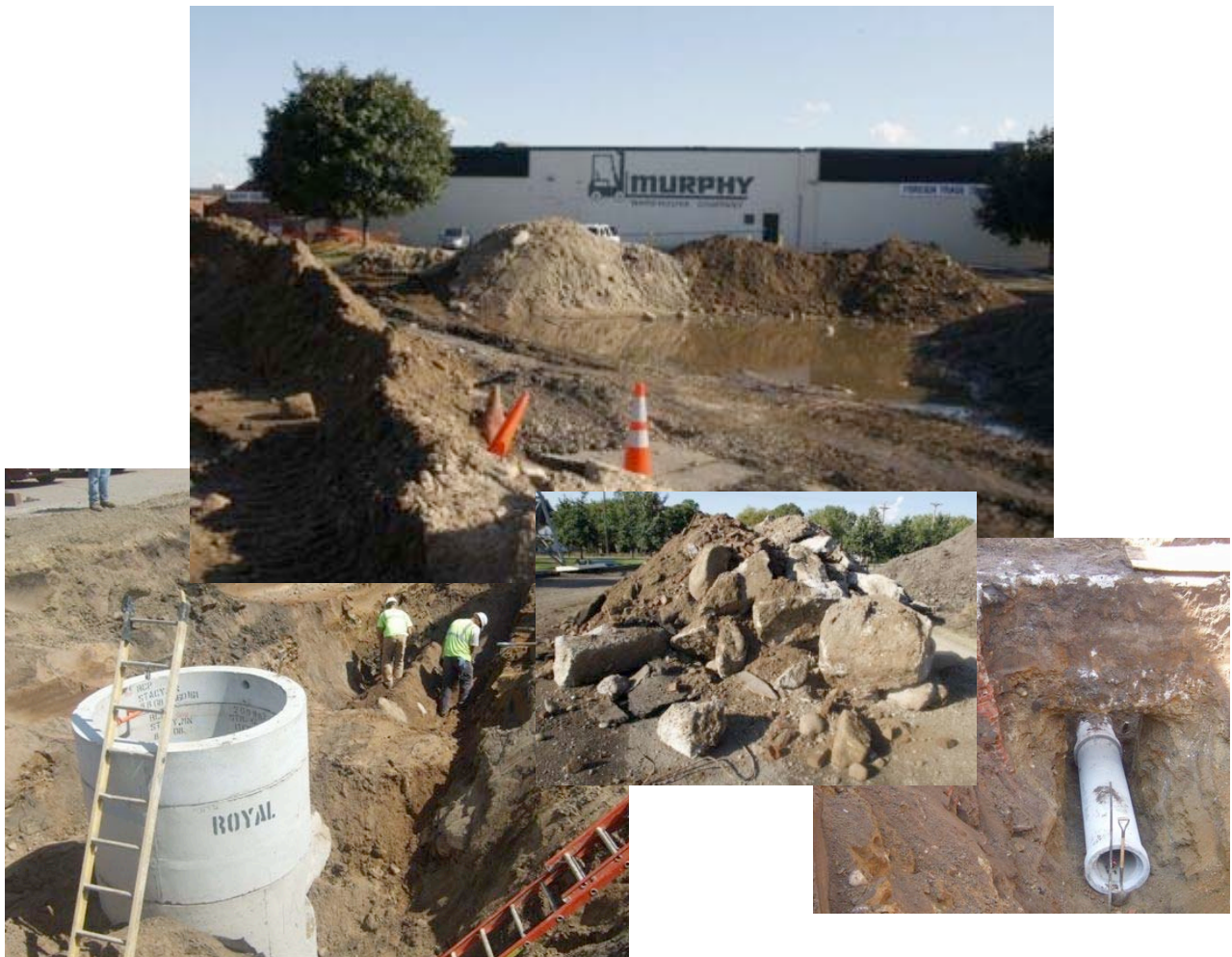
Photos are of stormwater management system construction at Murphy's Minneapolis facility
